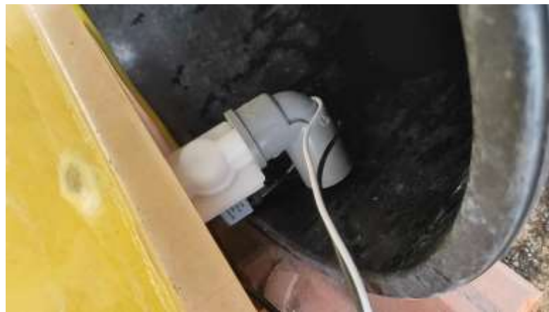
Gambar 5. 4 Actuator Pipa Solenoid
